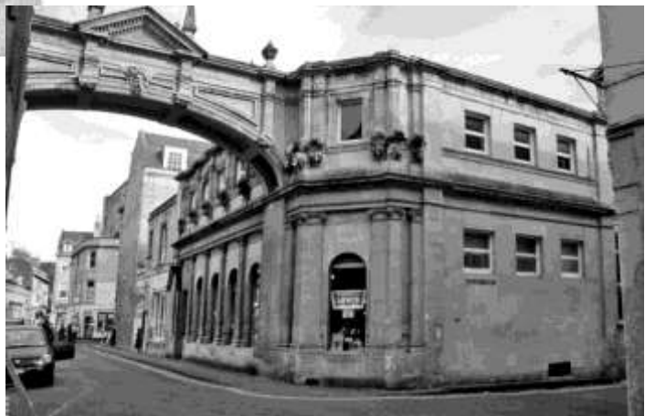
Archway and site of laundry >
